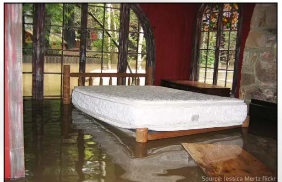
Flood, water damage, fire, etc.
